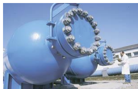
High pressure tanks 200 bar
